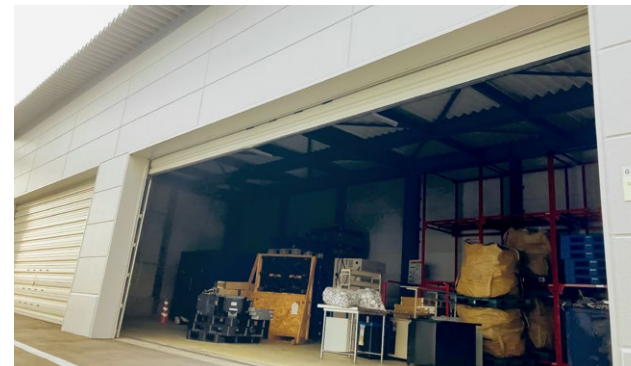
Recycling building at the Shiga Product Supply Center
